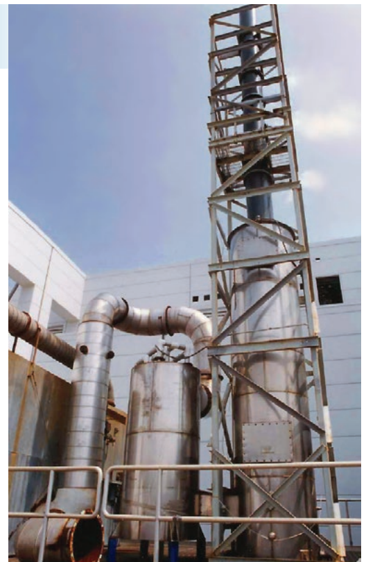
Packed tower and quench of high alloy for pharmaceutical industry.
