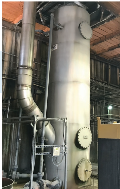
Packed tower for SO 2 absorption and neutralization for petrochemical industry.
