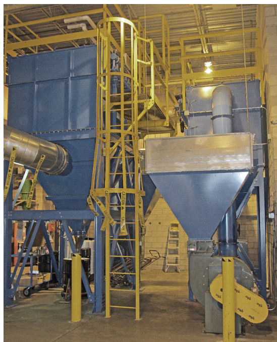
Sly's custom HEPA housing transition allowing safe recirculation of the filtered plant air.
