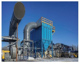
The bags in Sly's Tubejet collector operated for 22 total months of continuous use before a bag change was needed. The collector itself has been running smoothly since the summer of 2013 with excellent results.
