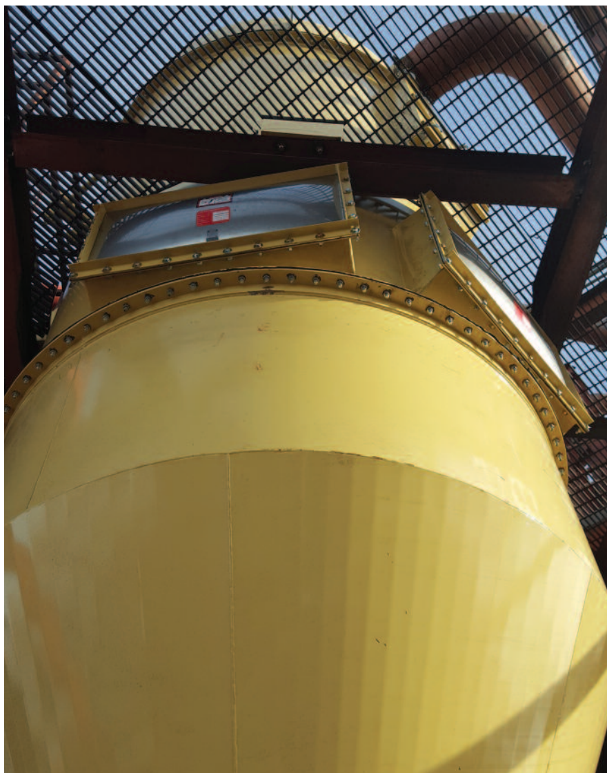
The new dust collector has an internal cyclone ring to help prevent wear.
