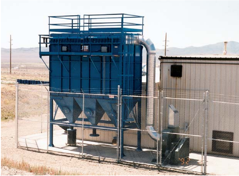
Conservative application of equipment and filter media results in high collection efficiencies. Continuous on-line cleaning is accomplished with low consumption of compressed air.
